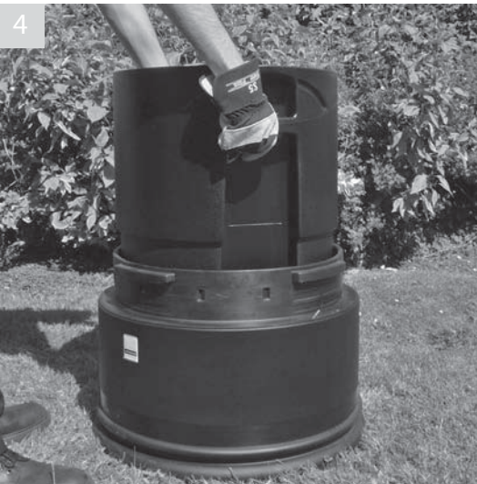
Grip liner using the two handles
