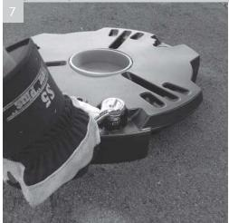
Use socket to tighten bolts, tighten to 22.0Nm torque for concrete. Tightening the bolts will fan out the bolt sheath holding the bolt secure: in the bin body, drop bin body to ground level
