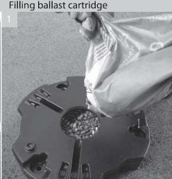
Remove cap and Pour gravel into the cartridge equally disperse gavel across the ballast cartridge fill to 30mm from top, replace cap
