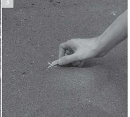
Remove ballast cartridge and clearly mark the ground in the three hole positions with a cross
