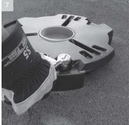
Use socket to tighten bolts, tighten to 22.0Nm torque for concrete. Tightening the bolts will fan out the bolt sheath holding the bolt secure
