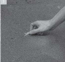
Remove ballast cartridge and clearly mark the ground in the three hole positions with a cross
