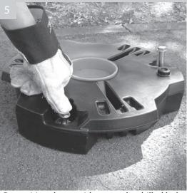
Drill 12mm holes in the three marked positions Re-position the cartridge over the drilled holes. Using a mallet drive bolts home Add washers to bolts and push through holes in cartridge locating into drilled ground holes
