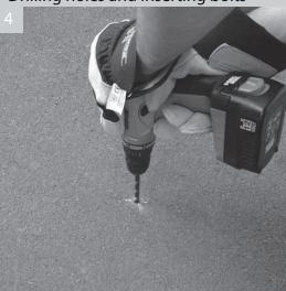
to a depth of 100mm to accommodate the bolt length, remove debris from holes
