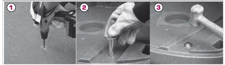
Drill 15 mm holes in the four marked positions to a depth of 110mm to accommodate the bolt length. Remove debris from the holes.
