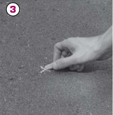
Move the bin to one side and clearly mark the ground in the four hole positions with a cross.
