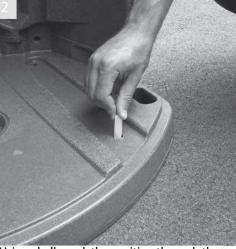
Using chalk mark the position through the four holes in the bin base onto the ground bellow
