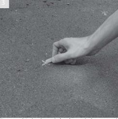
Remove bin body and clearly mark the ground in the four hole positions with a cross
