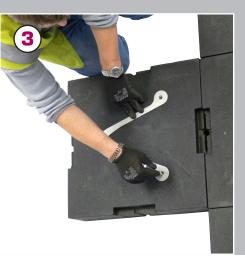
To insure the correct bin allignment, place the Using the plate as a guide drill 3 x 13mm holes Mark the position through the three holes onto the ground below using the bracket as a guide.
