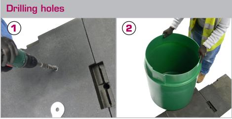
Drill 3 x 12mm holes in the ground to a depth of 100mm to accommodate the bolt length and remove debris from holes.
