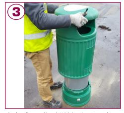
Replace liner and hood. With hood resting on base rotate hood clockwise until it will rotate no further. Push lock in to engage
