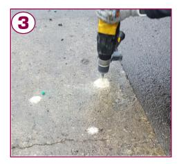
Drill 12mm holes in all 3 marked locations. Remove the debris from the holes.
