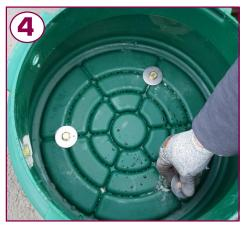
Re-position the bin over the drilled holes. Add washers to bolts and push through moulded holes locating into drilled ground holes beneath
