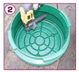
Turn the base over, remembering to position in the correct orientation. Use the masonry drill to drill though each location hole marking the ground.
