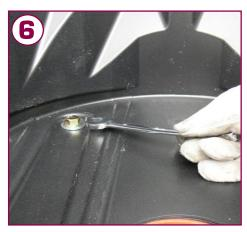
Tighten the bolts to 22.0Nm torque for concrete. Tightening the bolts will fan out the bolt sheath in the hole holding the bolt secure.
