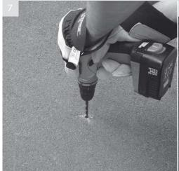
Drill 12mm holes in the four marked positions Replace bin locating over ground holes to a depth of 70mm to accommodate the full length of the bolts. Clear debris from holes
