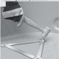
Put washers onto bolts. Push bolts into the three holes and drive them home with a hammer
