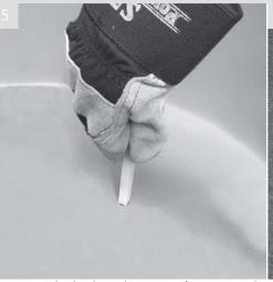
Position the body in the correct location and orientation. Mark through the holes in the base below in the three bolt locations to the ground below
