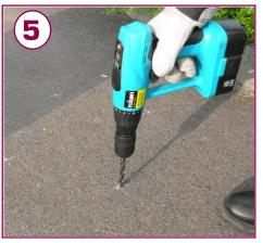
Drill 16mm (must be 16mm dia) holes in the four marked positions to the depth of 100 mm. Remove debris from holes.
