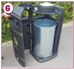
Re-position the bin over holes. Add washers to the bolts & push through moulded holes in bin base & into the drilled ground holes.
