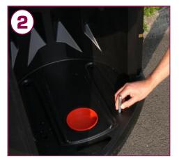
Using chalk, mark the position through the four holes in the bin base onto the ground bellow.
