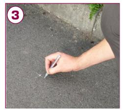
Remove bin body and clearly mark the ground in the four hole positions with a cross.
