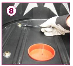
Tighten the bolts to no 22.0Nm torque for concrete. Tightening the bolts will fan out the bolt sheath in the hole holding the bolt secure.
