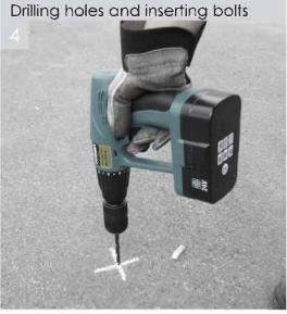
Drill 12mm holes at the four marked positions to a depth of 115mm to accommodate the ground fixing bolts.
