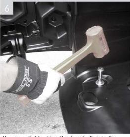
Use a mallet to drive the four bolts into the ground fixing holes, through the moulded holes in the base.
