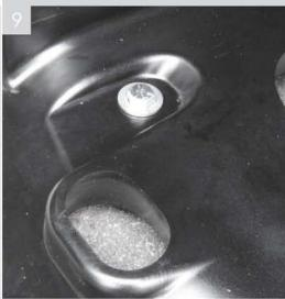
Tighten the bolts to 22.0Nm torque for concrete. Tightening the bolts will fan out the bolt sheath holding the bolt secure.
