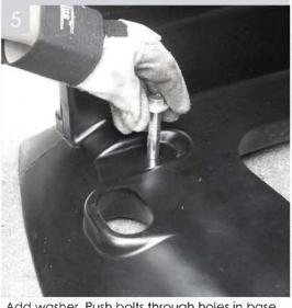
Add washer. Push bolts through holes in base locating into drilled ground holes.
