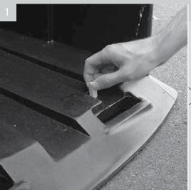
Position the body in the required location and orientation, mark through the holes in the base to the ground below
