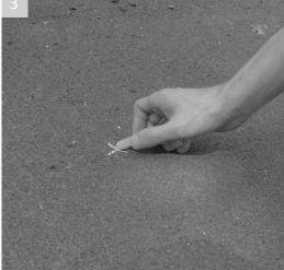
Remove the body to expose the ground below, clearly mark the positions of the four holes with a cross
