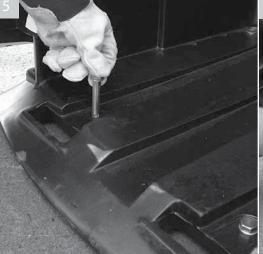
Add washer. Push bolts through holes in bin locating into drilled ground holes
