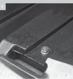
Tighten the bolts to 22.0Nm torque for concrete. Tightening the bolts will fan out the bolt sheath in the hole holding the bolt secure
