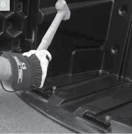
Use a mallet to drive the four bolts into the holes drilled in the ground through the moulded holes in the bin base
