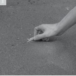
Remove the body to expose the ground below, clearly mark the positions of the four holes with a cross
