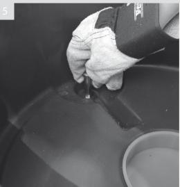
Drill 12mm holes in the three marked positions Re-position the base over the drilled holes. Add Using a mallet drive the bolts home washers to bolts and push through moulded holes in base locating into drilled ground holes
